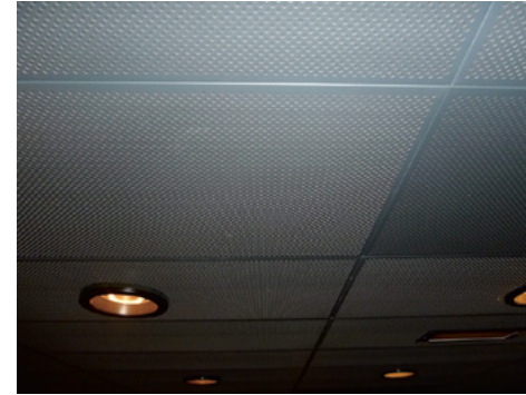
► Black ceiling in a cinema with visible grid.
